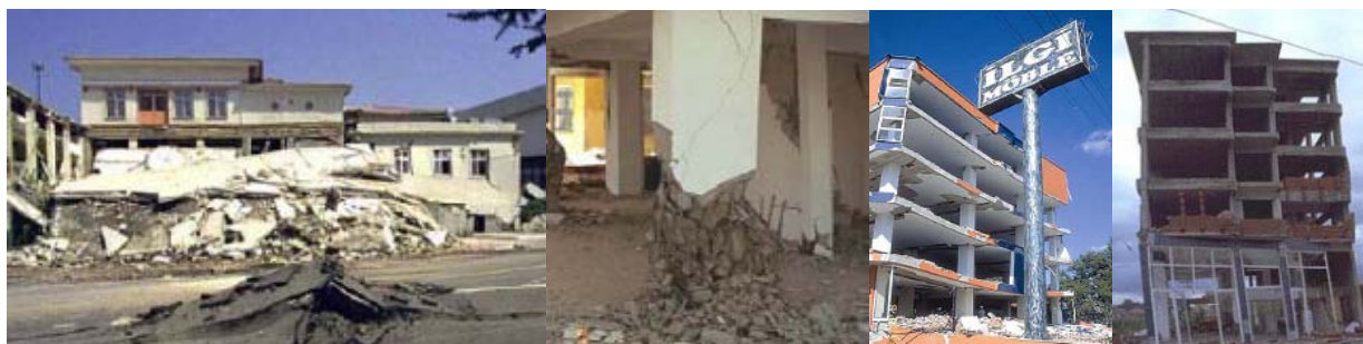
Figure 1: Building damage from the November 1999, Ms=7.2 earthquake (PEER, 2000).
