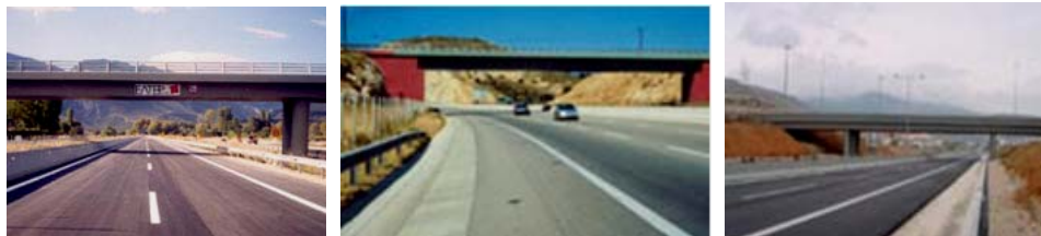
Figure 3 Typical bridge overcrossings in Greece
