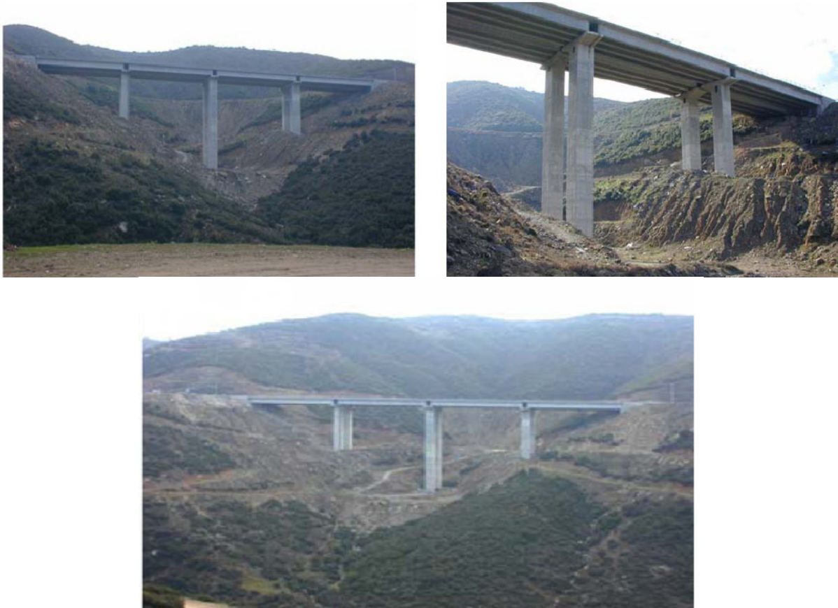
Figure 1: General overviews of the 2 nd Kavala Ravine Bypass Bridge.
