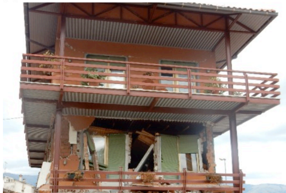
Figure 8. Steel residential building (a) after the first earthquake and (b) after the entire sequence. (a) Limited non-structural damage and (d) complete non-structural damage at ground level with consequent residual drift.
