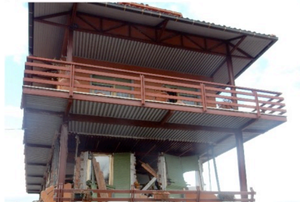
Figure 8. Steel residential building (a) after the first earthquake and (b) after the entire sequence. (a) Limited non-structural damage and (d) complete non-structural damage at ground level with consequent residual drift.
