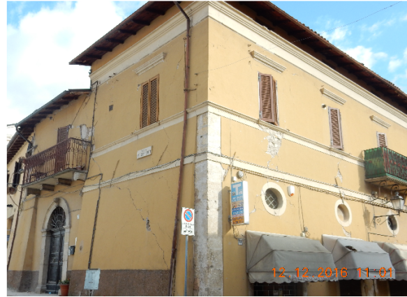
Figure 7. Masonry residential building (a) after the first earthquake and (c) after the entire sequence.
