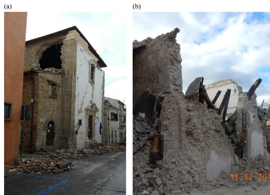
Figure 6. Masonry church in Amatrice after the (a) first and (b) second survey.
