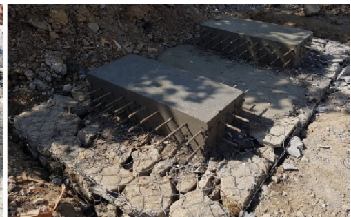
Figure 7 Cross section of the RC pedestal (left); Laid rebar before casting (mid); Casted RC Pedestals (right)
