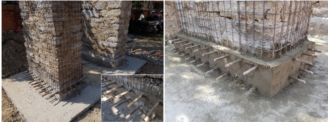
Figure 8 Wire mesh tied and welded to the rebar of the pedestal (left); Connections covered with 50mm of 1:6 plaster (right)
