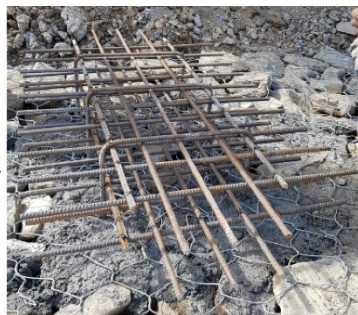
Figure 7 Cross section of the RC pedestal (left); Laid rebar before casting (mid); Casted RC Pedestals (right)
