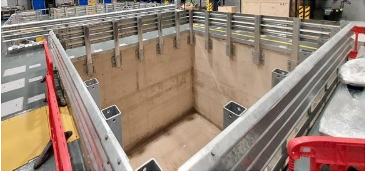
Figure 3. Photo of the 6m x 5m test pit with a 4-meter depth.
