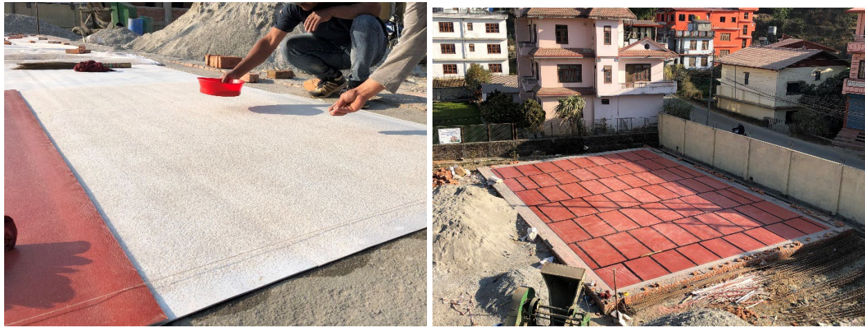
Figure 4.2 Spreading of the sand across the PVC surface (left) and PVC-s isolation (right).
