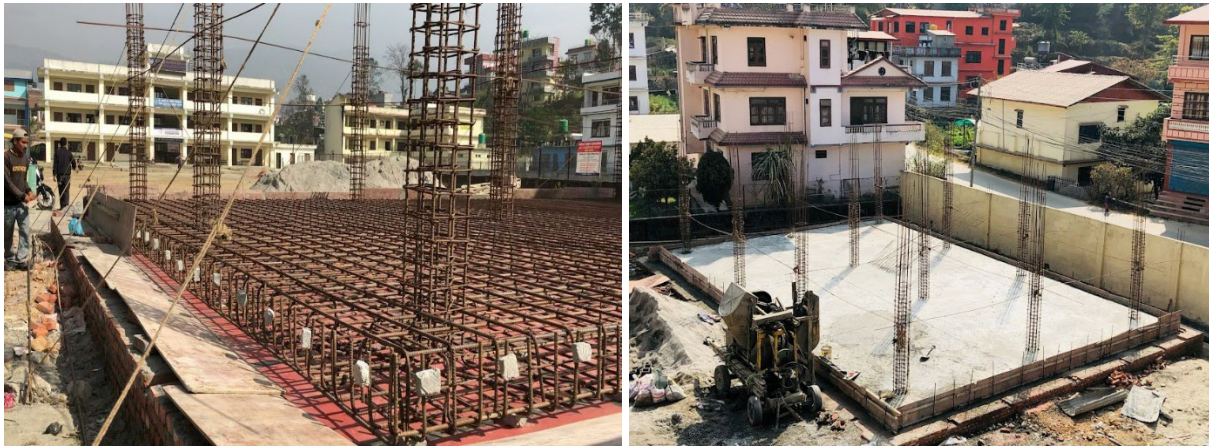
Figure 4.3 Overview of the mat foundation construction.
