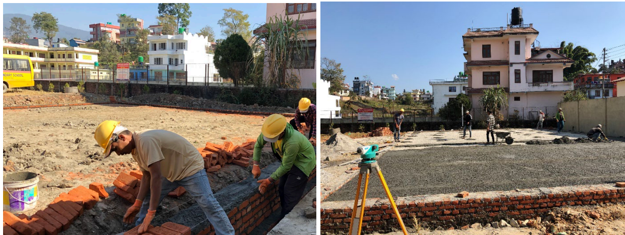
Figure 4.1 Construction of the sacrificial parapet (left) and surface leveling (right).
